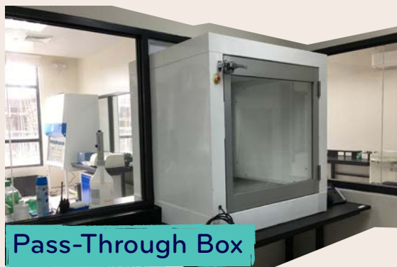
Figure 2. Pass-through box as seen from the record section of the COVID-19 laboratory passing into the RNA Extraction area. The latter is the "dirtiest" section of the laboratory where actual processing of potentially virus-containing samples occur. A safety lock mechanism is also installed preventing simultaneous opening of both sides of the pass-through box during operation.
